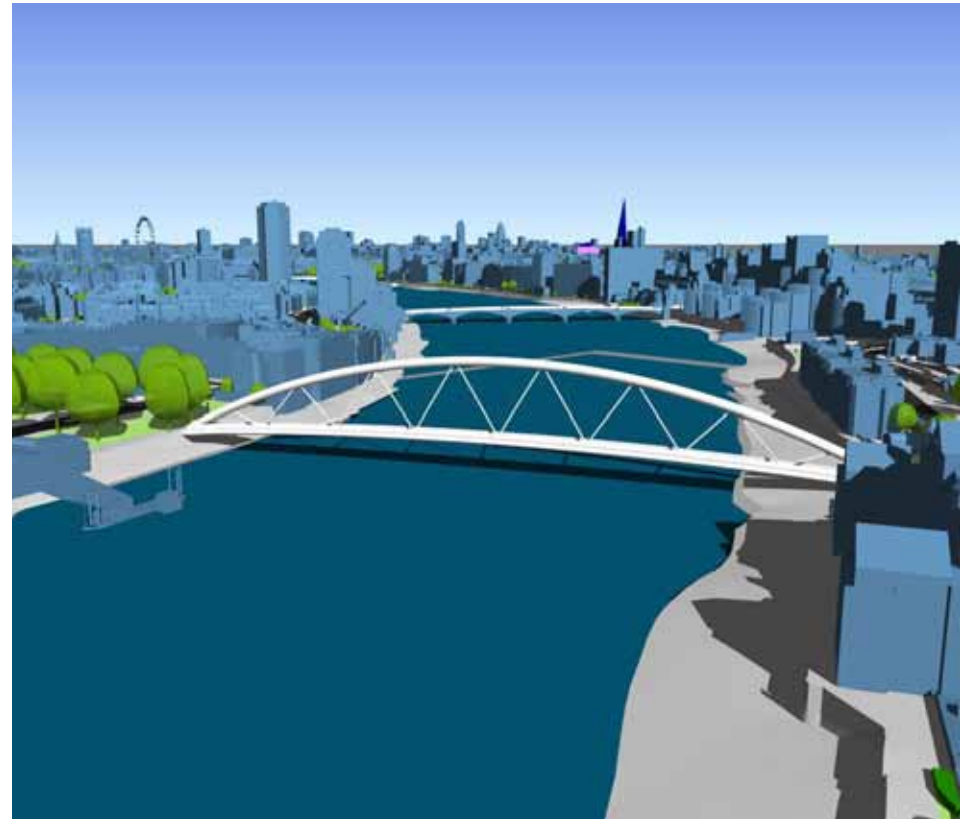
Figure 7.38 bridge type 3 from above Nine Elms Pier
